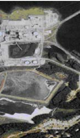
Coal Fired Plant.
